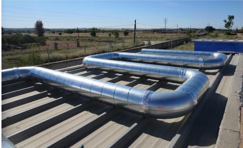
**Figure 11:** Final scheme of ducts installation
