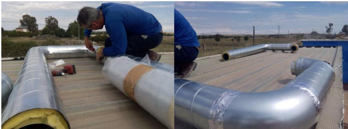
**Figure 10:** Works on rooftop (Reference bends & pipes)
