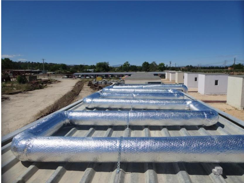
**Figure 15:** Works on rooftop (NANOHVAC bends & pipes). Finishing touch
