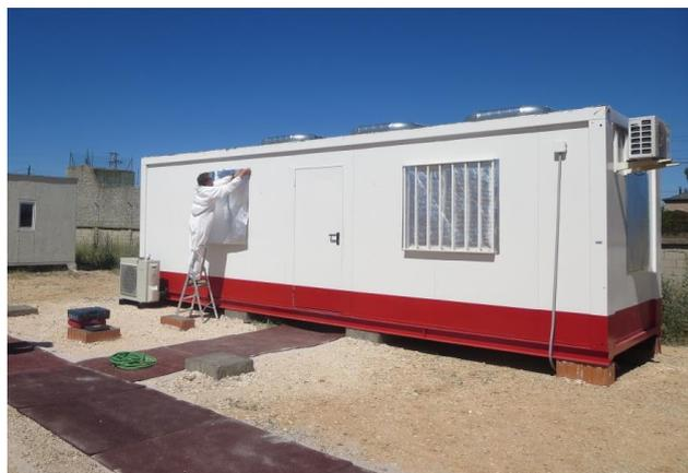
**Figure 19:** Western and Southern windows were blocked to diminish thermal load and solar gains (Northern window remained diaphanous)
