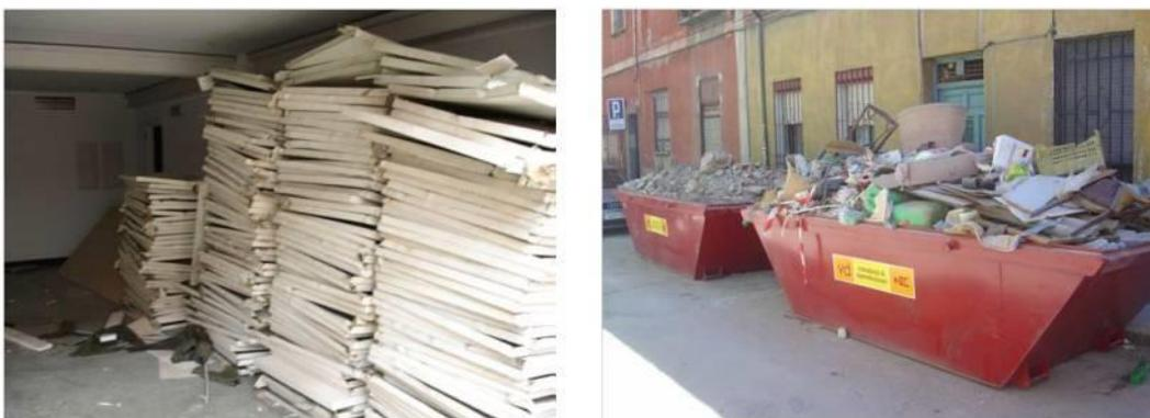
**Figure 33.** Panels separated from other demolition or refurbishing residues (left) and a mixture of residues that are part of the CDW (right)
