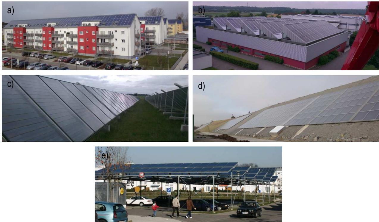
**Figure 3: a) Renovated multi-family houses with retrofitted solar thermal collectors in Crailsheim/Germany; b) Gymnasium in Eggenstein/Germany; c) Ground mounted collectors in Jægerspris/Denmark; d) Collectors on noise barrier wall in Crailsheim/Germany; e) Collectors as “carport” in Neckarsulm/Germany (source: University of Stuttgart)**
