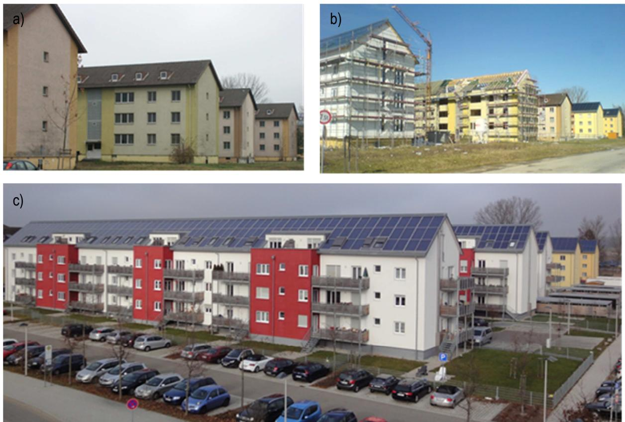
Figure 8: a) former military buildings before retrofitting; b) during retrofitting; c) completely finished (source: University of Stuttgart)
