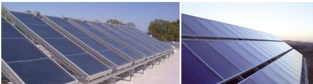
**Figure 7: Settings of Large-format flat plate collectors, either horizontal or vertical alignment**
