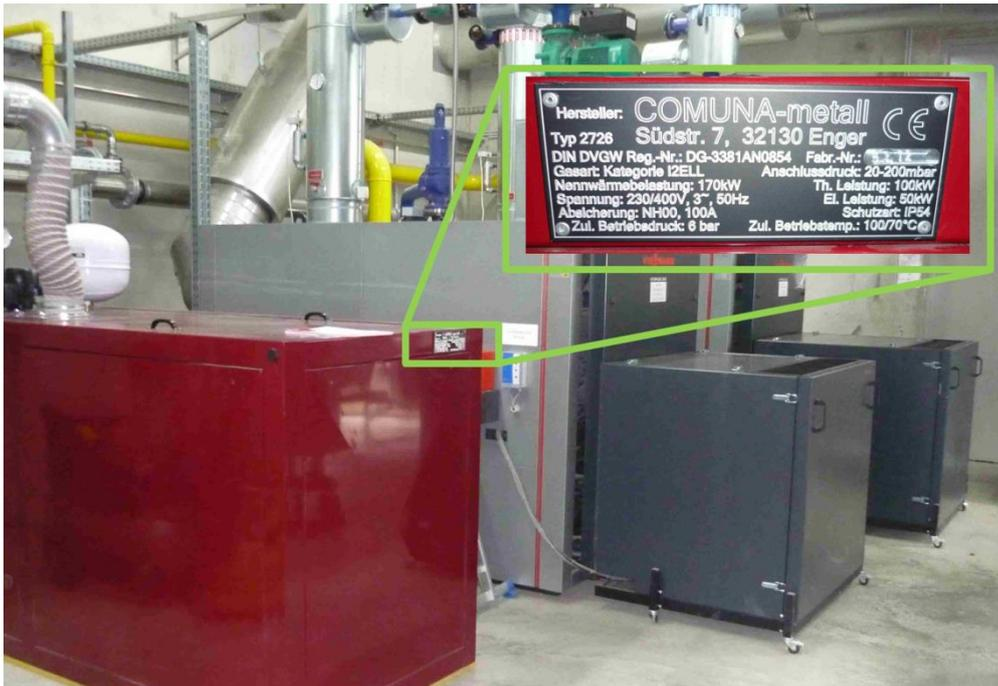
Figure 12 CHP with rating plate
