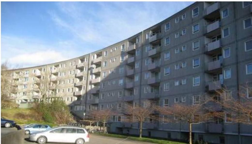
Figure 3: A typical house with prefabricated elements and visible joints from the post-war era.
