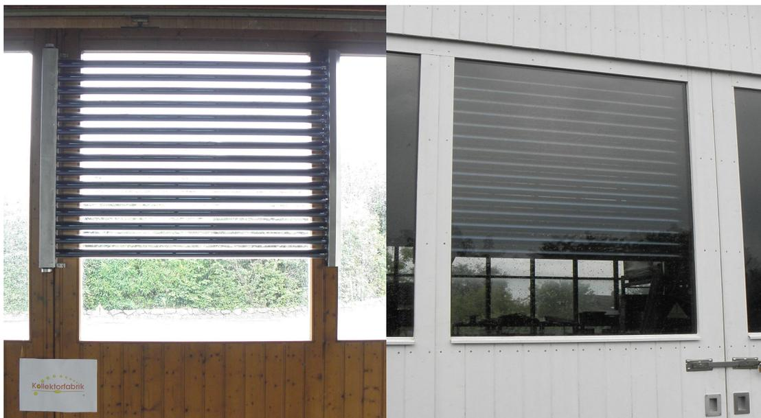
Picture 3: New Cost-Effective collector prototype mounted at the windows of our Kollektorfabrik storehouse
