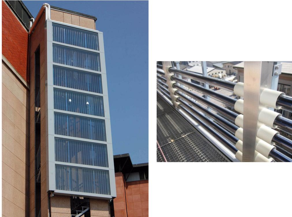
Figure 10 pilot installation in the Slovenian pilot building in Ljubljana. Air heating vacuum tube collectors (right) and transparent solar thermal collectors (left) are used for solar heating and cooling.
