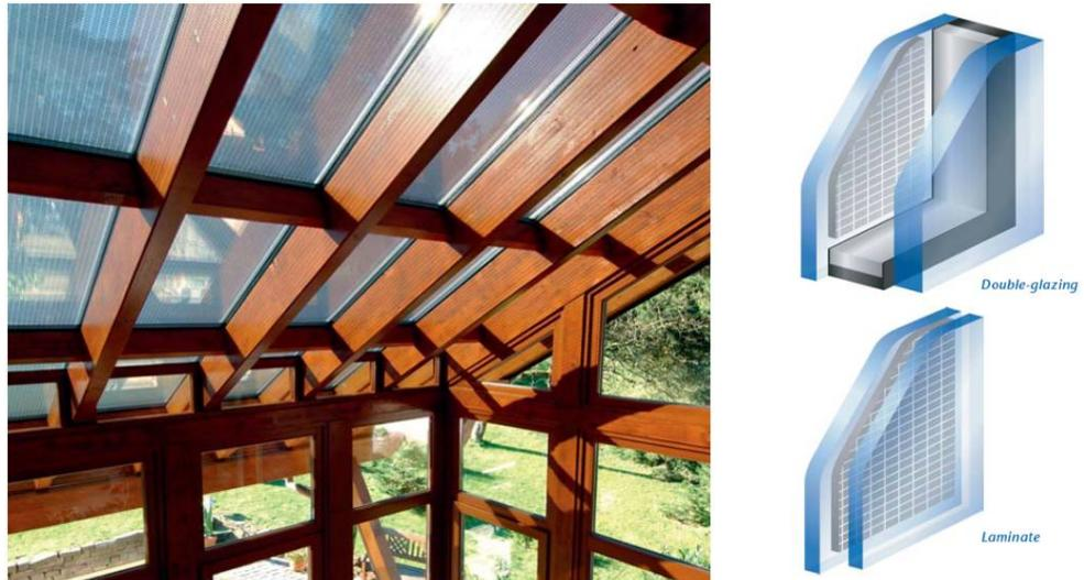
Figure 24: The picture on the left shows an example of roof integration. On the right two different solutions for ASI technology (Source: SCHOTT).
