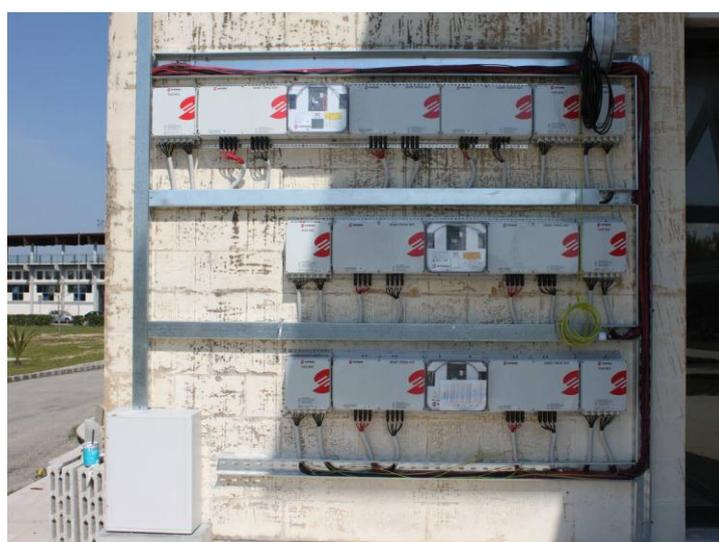
**Figure 58 – smart string of the photovoltaic roof on “Museo dell’ambiente”**
